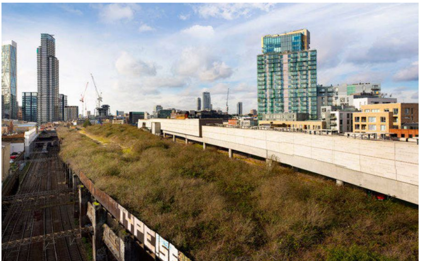
Figure 8: Existing photograph of platform level above Braithwaite Viaduct from the east end of site looking west.
