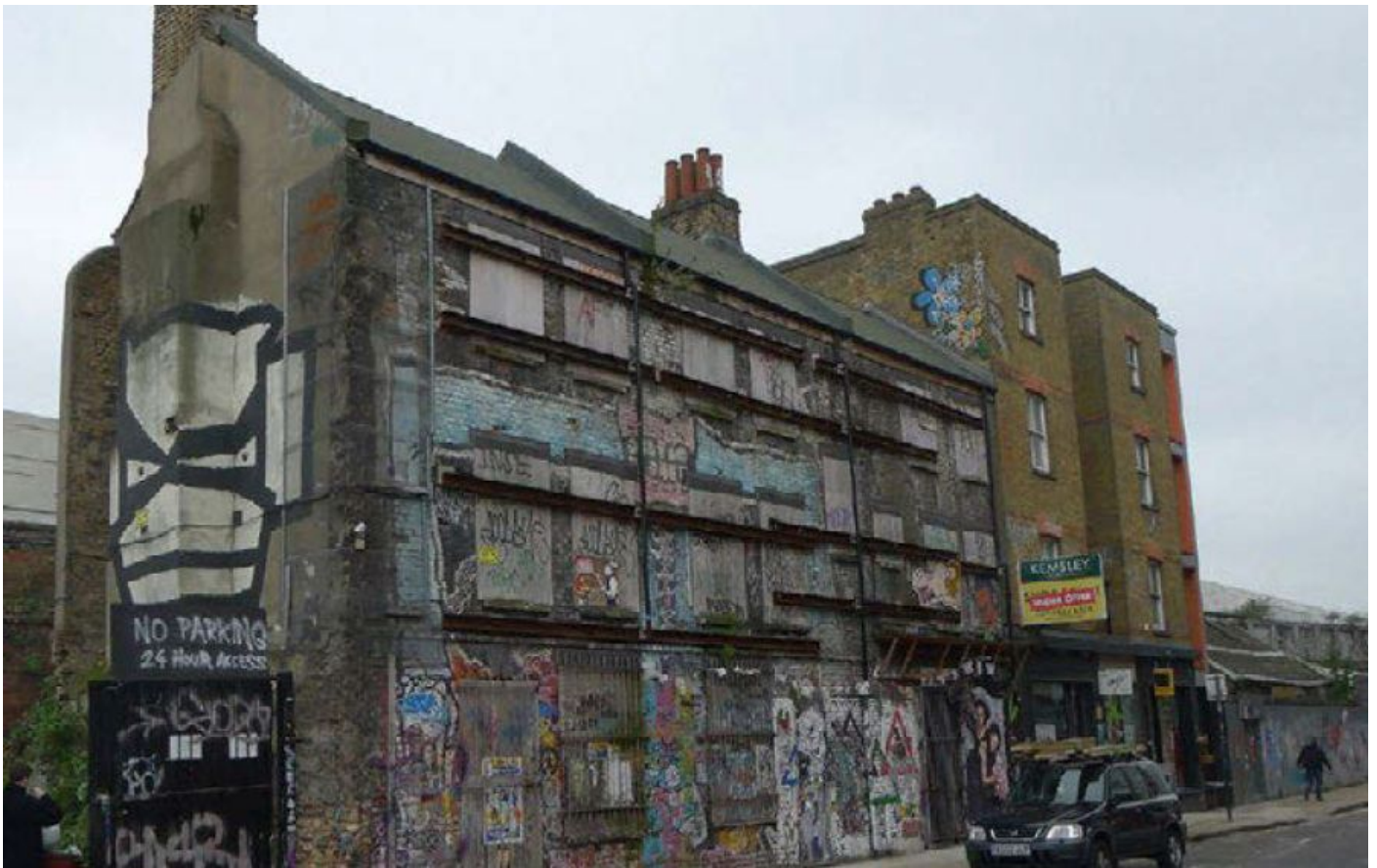
Figure 15: Sclater Street buildings
